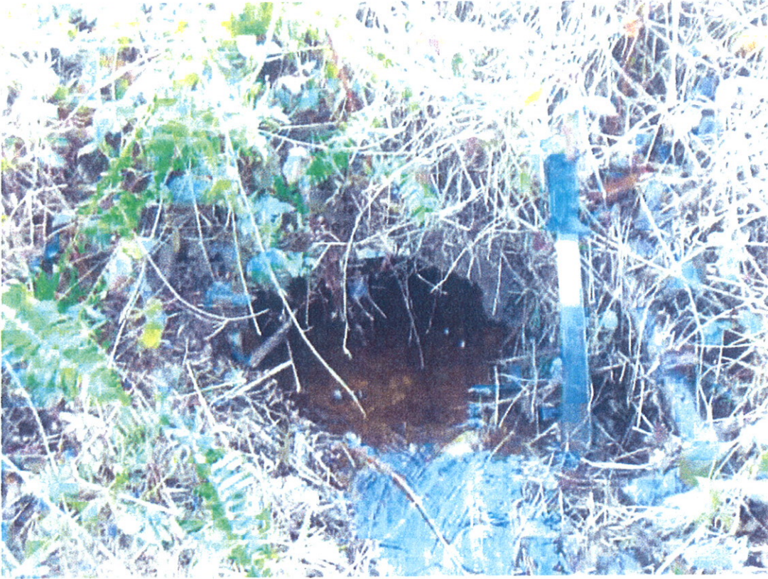
CONSTANCE DR. CULVERT CROSSING
