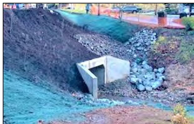
Ostrich Creek at Kitsap Way, after construction.
