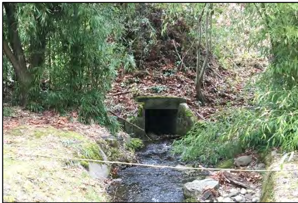
Ostrich Creek at Kitsap Way, pre-construction.
