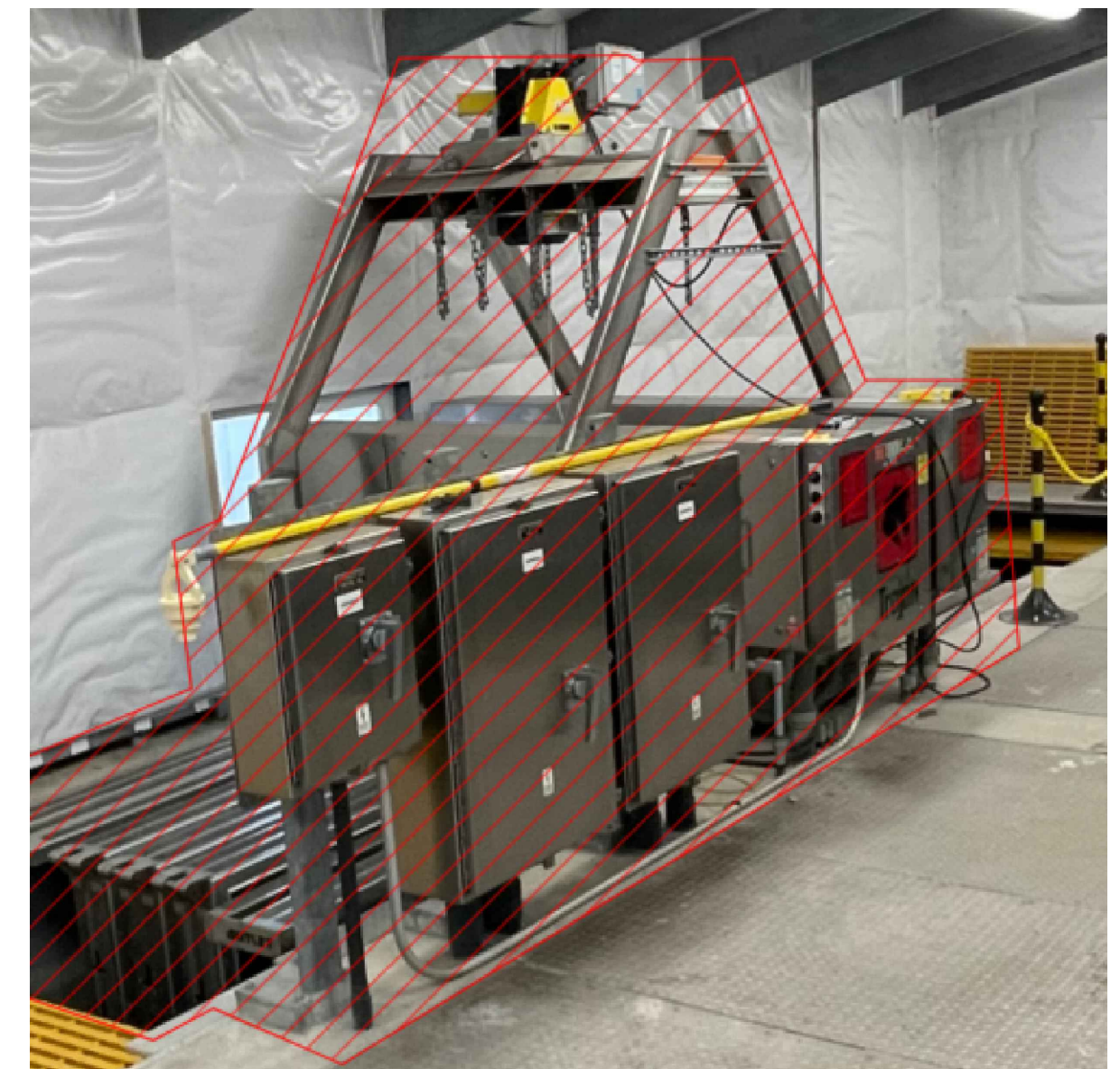
EXISTING UV4000 SYSTEM DEMOLITION
