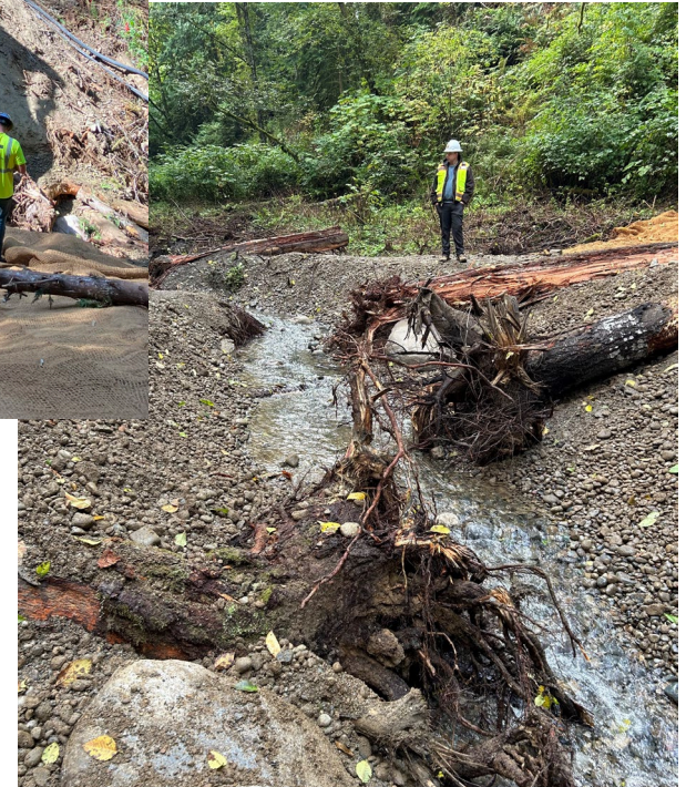
East Fork Restored
