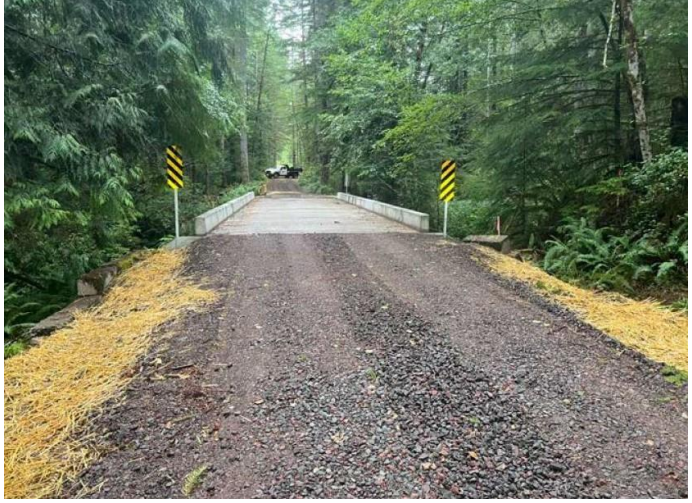
Photo 2. Railcar Bridge Replacement
