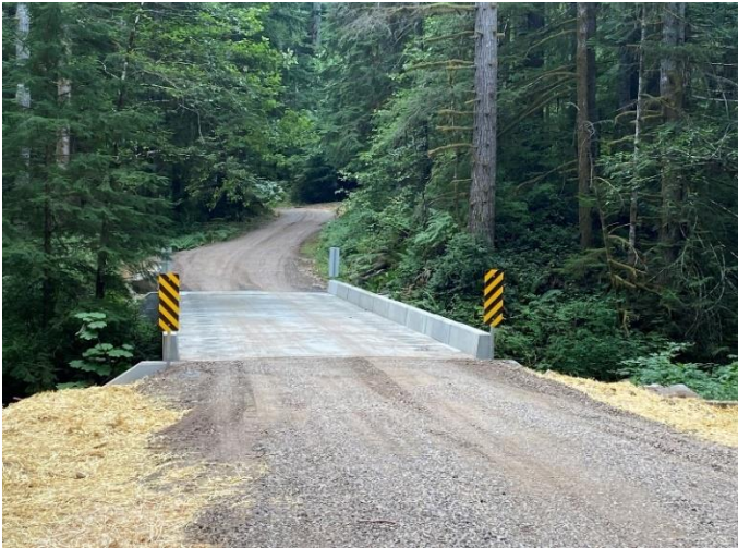
Photo 3. Vessey Bridge Replacement
