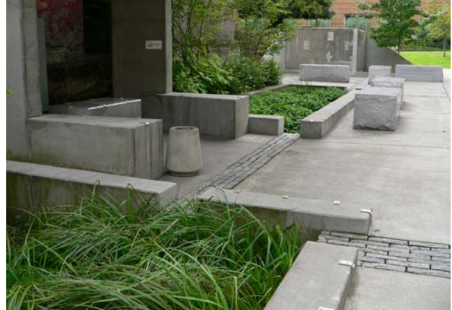
Bioretention planters. figure 6.1.7 Source: Curtis Hinman
