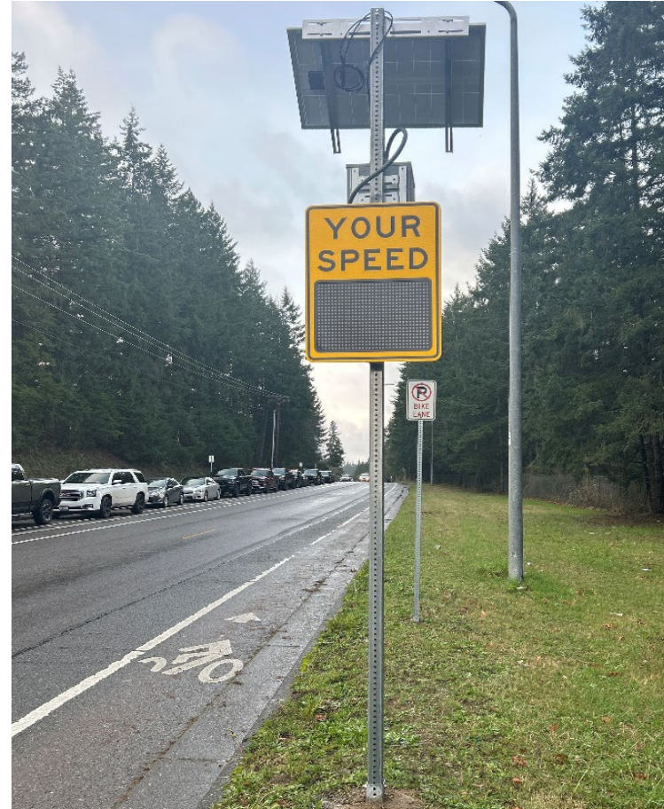
Speed feedback sign installed near John D. “Bud” Hawk Elementary School
