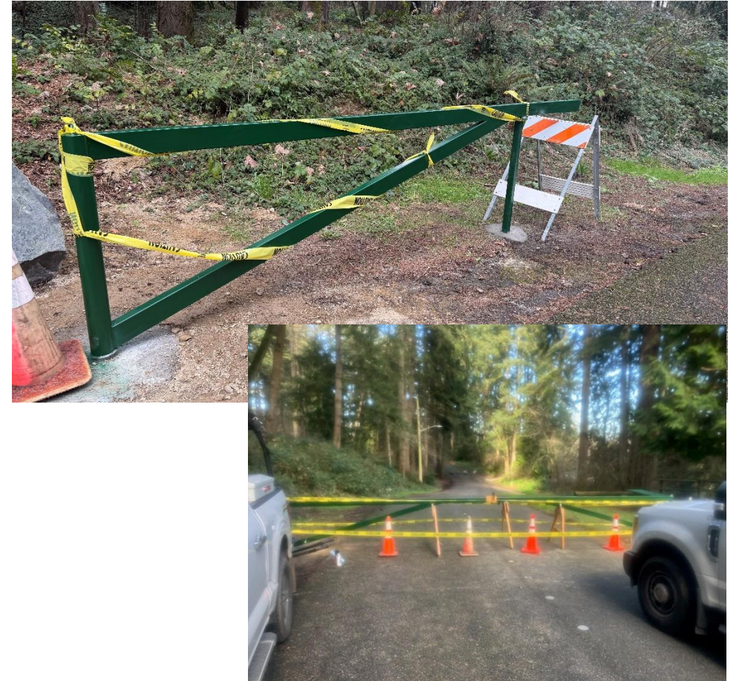
New Gate Installation at Forest Ridge Park photos taken on Mar. 3, 2026
