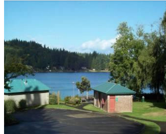
Price Road Pump Station – Kitsap Lake Park
