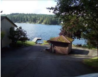
Chico Way Pump Station
