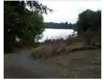
Root Court Pump Station
