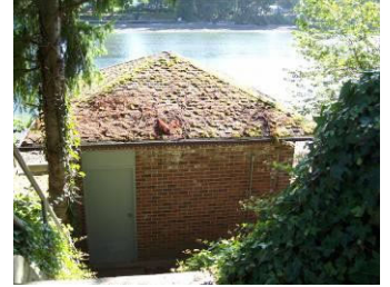
Madrona Point Alleys East Pump Station (The Crossing)
