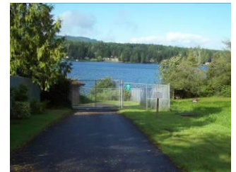
Cedarwood Drive Pump Station
