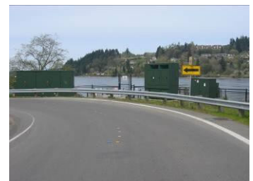
Snyder Avenue Pump Station
