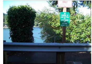
Madrona Point Alleys West Pump Station (The Crossing)
