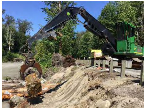
SR 530 bank stabilization, south of Rockport, in August 2019
