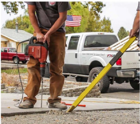
Sidewalk Slab Raising
