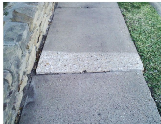
Sidewalk Grinding
